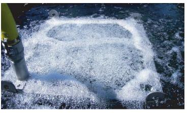
JAEGER BioCube<sup>TM</sup> a Self-weighted Retrievable fixed film stationary media module pre-engineered as a high rate air-lift reactor for enhanced BOD and/or Ammonia removal. JAEGER BioCube™ consist of a vertical channel biofilm support media in honeycomb arrangement combined with JAEGER OxyStrip™ strip diffusers for optimized air supply and uniform scouring of excess biomass.
