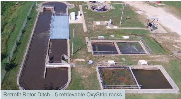
Retrofit Rotor Ditch - 5 retrievable OxyStrip racks
