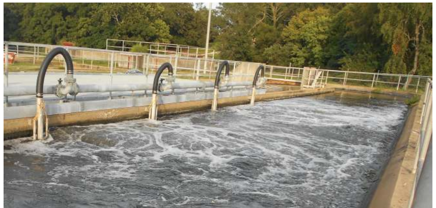
Single Train WWTP - 26 retrievable OxyStrip racks
